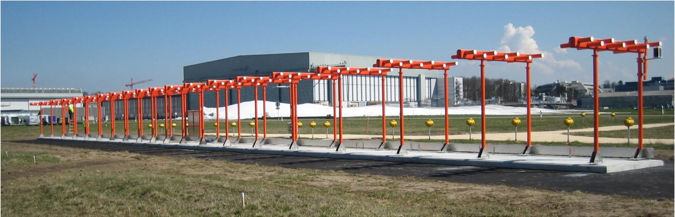
**Figure 3: Reduced Coverage Localizer Installation at Zurich Airport**
